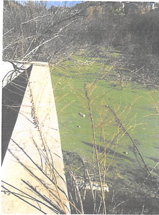
Partially blocked drain at downstream portion of Greer Rd. near Nutmeg St; photo taken 12/15/2017 by SAWA.
