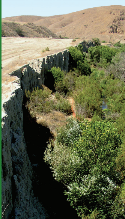
Temescal Wash suffered massive erosion from its banks, leaving a verticle cliff.
